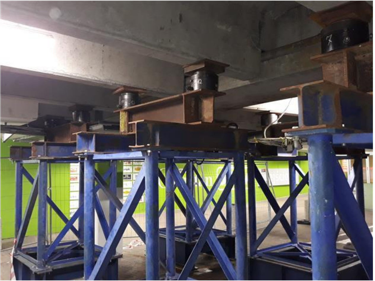
Lifting up the slab structure
