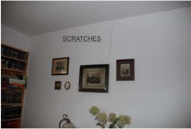
Partition walls - damages (scratches) and restoration.
